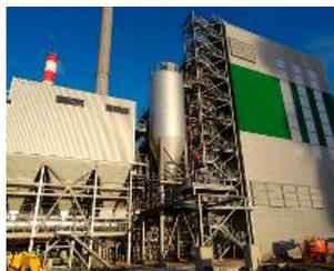
The Biolaq Energies project, in Lacq, is a biomass-fired CHP plant of 54 MW, that utilises forestry wood, and clean, uncontaminated residues from wood processing.
