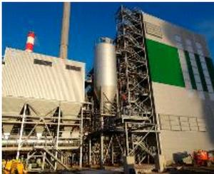
The Biolacq Energies project, in Lacq, is a biomass-fired CHP plant of 54 MW, that utilises forestry wood, and clean, uncontaminated residues from wood processing.
