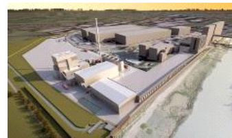
Tilbury Green Energy Plant - a 40 MWe power plant close to London, is to be delivered by AET.
