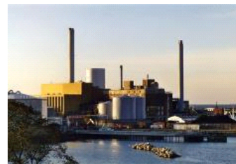
Coal to biomass conversion at Østkraft.
