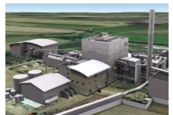
The JG Pears plant will be using MBM and woodchips as fuel.
