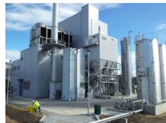
The Rothes CoRDe biomass-fired CHP plant off to a successful start.
