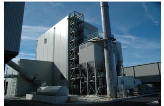
Western Wood Energy Plant has a net efficiency of 30%, - even though designed back in 2005.
