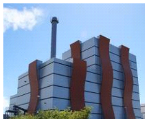
The SODC Orléans cogeneration plant supplies district heating to 15,000 homes, equivalent to 27% of the city of Orléans.
