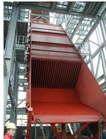
Installation of boiler super heater section
