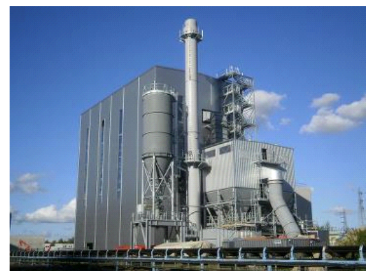
Cofely Services - Bio Cogelyo Normandie (BCN) in France is a biomass-fired cogeneration plant with an annual fuel input of 165,000 tons of biomass fuel.
