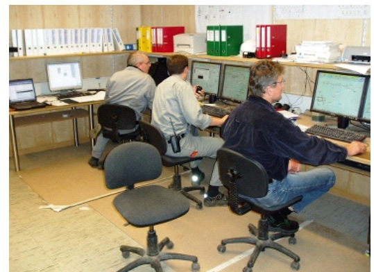
AET monitors and analyses the plant and proposes possible improvements to be made
