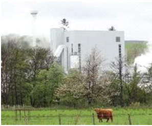
Rothes CoRDe Ltd is a biomass-fired cogeneration plant in Scotland fuelled by a whisky by-product and clean wood.
