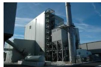
The biomass power plant has a 48MW<sub>th</sub> Biomass Boiler with the newest [AET Combustion System](#) which fulfils stringent emission criteria without the use of SNCR and lime.
