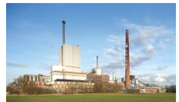
The Solvay plant in Rheinberg.
