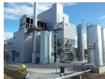
The Roths CoRDe cogeneration plant produces heat and power.
