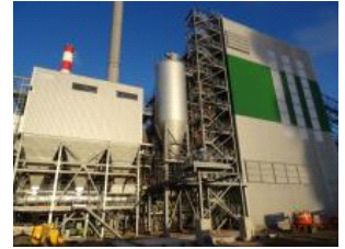
The Biolacq Energies project, in Lacq, is a biomass-fired CHP plant of 54 MW, that utilises forestry wood, and clean, uncontaminated residues from wood processing.
