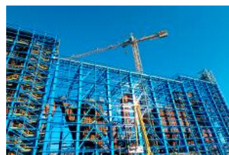
Boiler and steel structure under erection.
