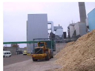
Linz-Mitte Energie Anlage in Austria - uses uncontaminated wood as fuel.
