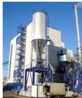
The FunderMax Biomasse Energieanlage is a biomass-fired combined heat and power (CHP) plant in Neudörfel, Austria.
