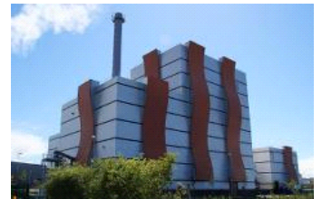
The biomassfired CHP plant in Orléans was commissioned in 2015.
