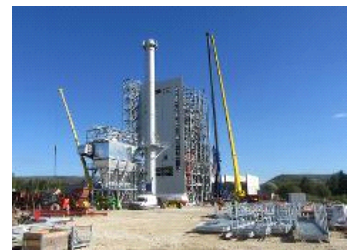
The plant is under construction (OCT 2017).
