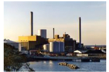
The CHP plant Østkraft was converted to be able to use 100% biomass in 2016.
