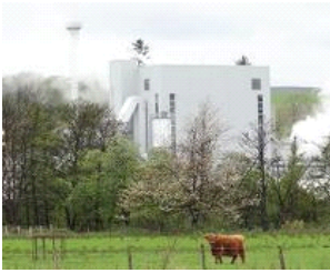
Rothes CoRDe Ltd is a biomass-fired cogeneration plant in Scotland fuelled by a whisky by-product and clean wood.
