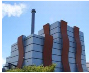
The SODC Orléans cogeneration plant supplies district heating to 15,000 homes, equivalent to 27% of the city of Orléans.
