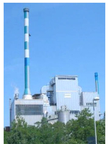
The Boehringer-Ingelheim CHP plant in Germany.
