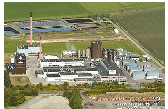
De Danske Gærfabrikker (DDG) reduced the NO x emissions by approx. 50% by using AET SNCR DeNOx System.
