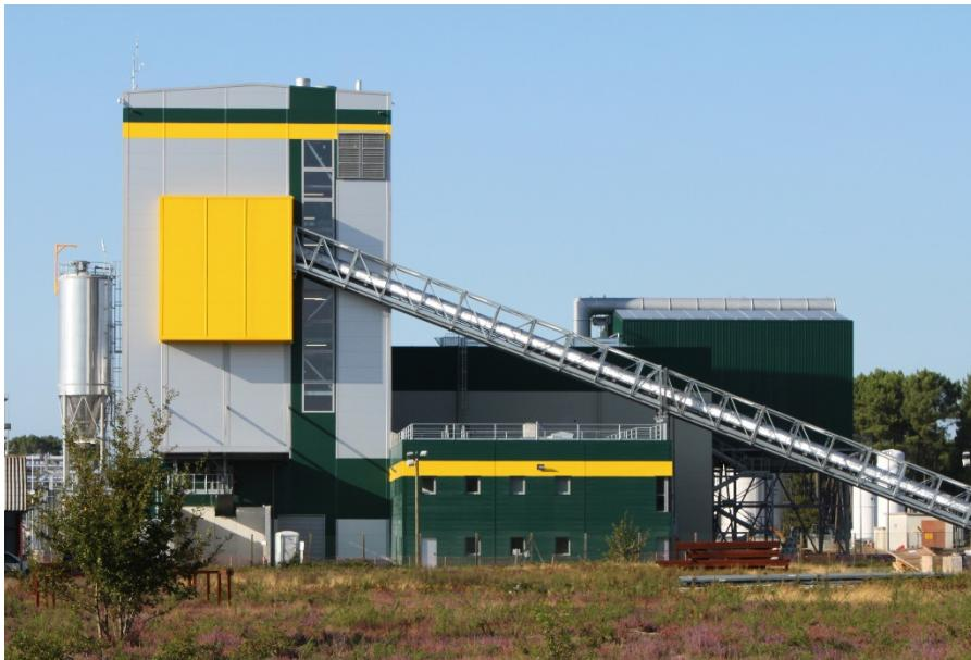
*The Biomass Energy Solutions VSG plant at the DRT site in Vielle-Saint-Girons is now in operation. The tested performances are well within the guaranteed values. The boiler efficiency is approximately 93%.*
