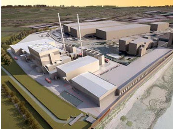
Tilbury Green Power, London, UK
